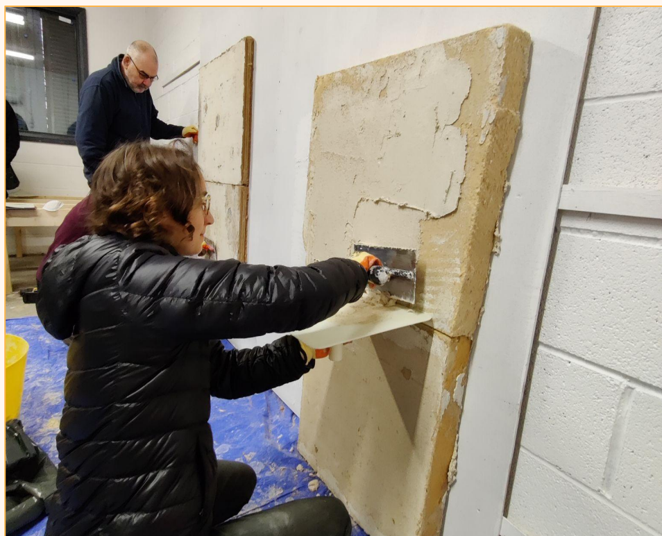
Using lime renders and plasters and insulation materials like woodfibre boards needs different skills to more standard drylining used in modern buildings - so training can be provided.
