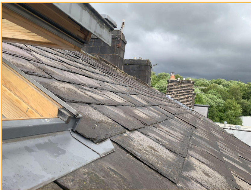
Roofs on back to back homes are shared with neighbours on either side and also to the rear. This can add complexity to retrofit projects - especially where roofs feature dormers and rooflights.
