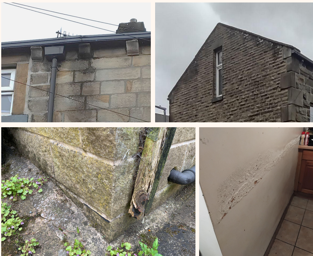
Images clockwise from top left: 1. A gutter joint with a leak where a new and old gutter meet, causing dampness in the stone wall. 2. A clipped verge - the edge of a roof at the gable - showing staining where wind driven rain is making the wall damp. 3. Evidence of high levels of moisture in walls at ground level where rain hits paved areas and bounces up onto walls. 4. Areas of damp on internal walls caused by poor drainage at ground level where walls are partially against the ground.
